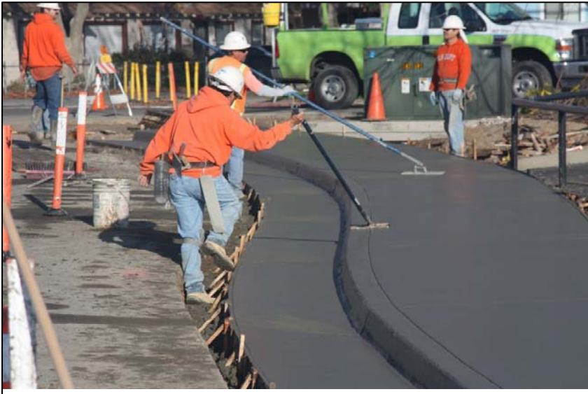
Construction on Riverside Avenue
